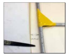
Fig. 4: Fabric can be pre-trimmed to match the tube size by using a little math—add tube diameter x pi x 0.8 to the perimeter line.
