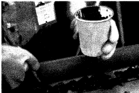
Fig. 14 Application of Brushable Sealants
